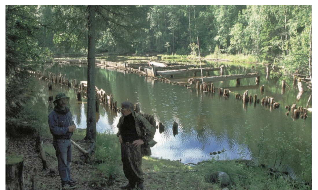
One of the wharfs used by boats transporting stone.
